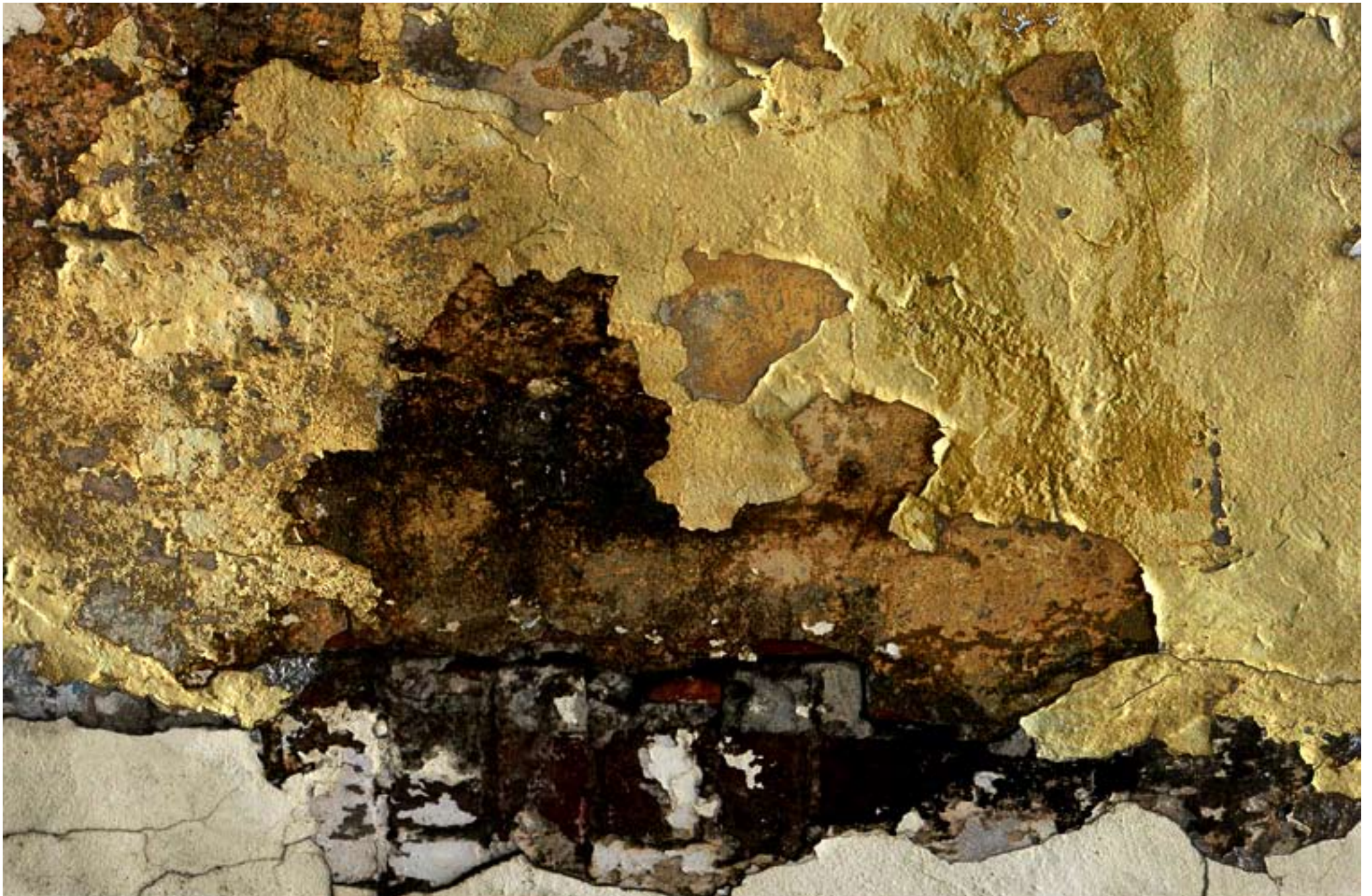
WALL AT GULGONG
