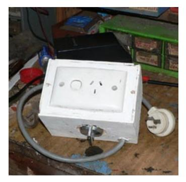
I made this timing mechanism for forgetful people who forget to switch the heater off in the bathroom. It consists of a timer out of an old washing machine that's timed to run for an hour to do the washing. I simply wired that inside an ordinary power outlet switch so that when you want to have a bath – say you're going to be twenty minutes. You plug the power into the socket, put the switch
