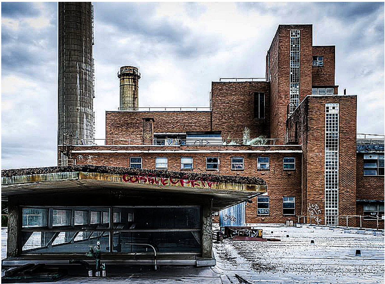
Administration building rooftop
