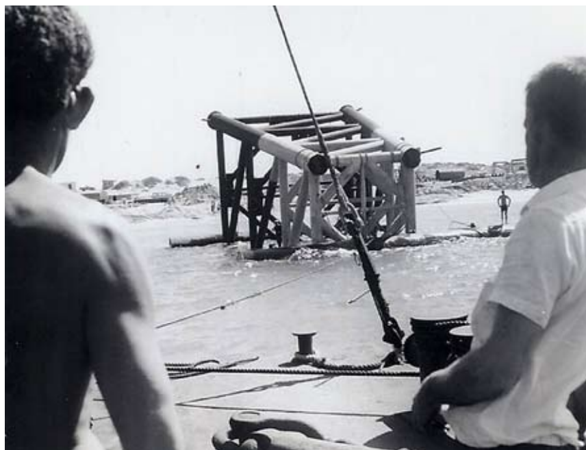
Positioning the towers
