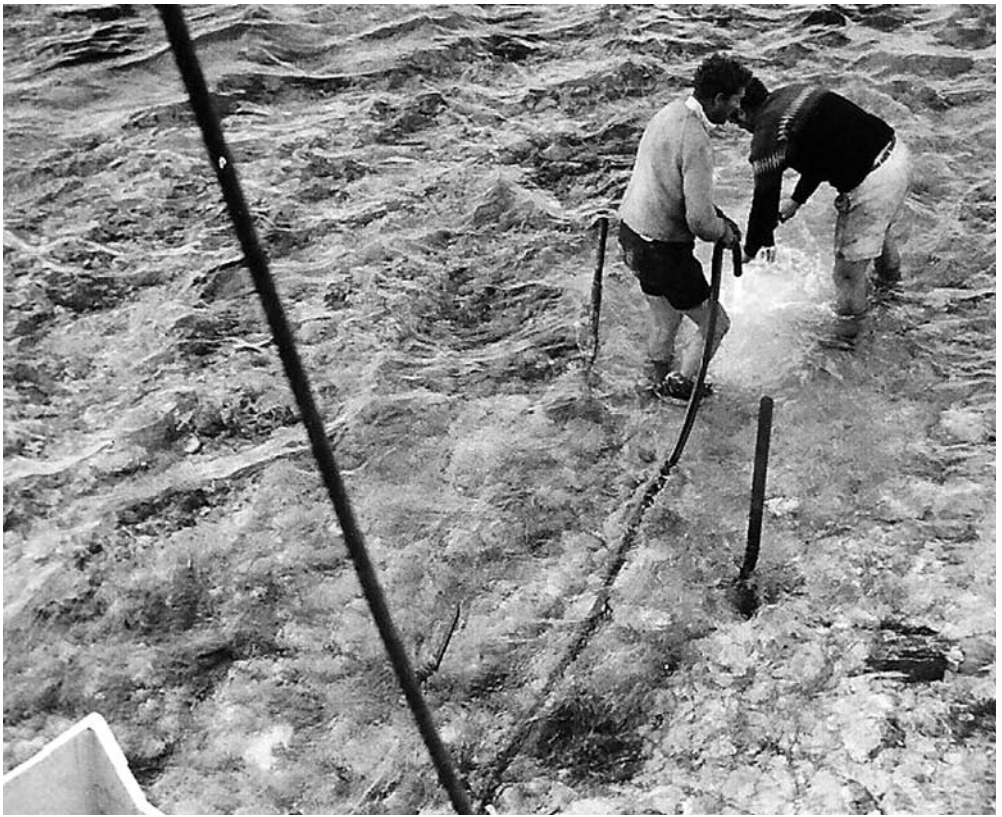
Drilling shot holes in the coral prior to blasting a passage to clear the Kinei Maru
